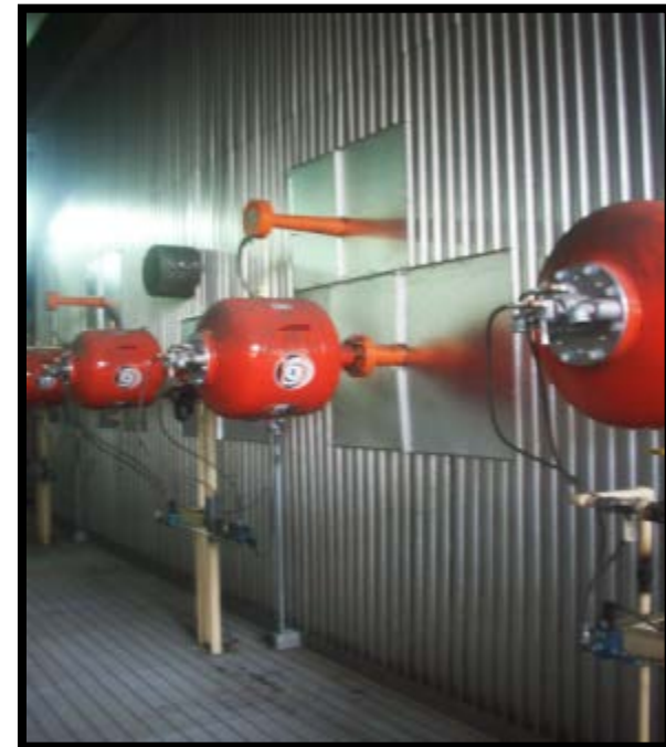
Ash Sweeper/Acoustic Cleaner Installation
