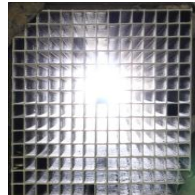
After Ice Blasting
