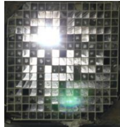
Before Ice Blasting
