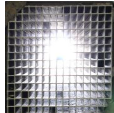
After Ice Blasting
